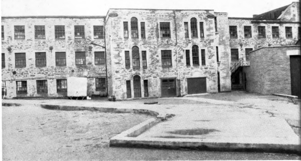
Page 72 (above) The cut-down remains of No 1 mill, the oldest surviving built by Dale c1786; (below) the north front of No 2 mill reconstructed c1905. Note the contrast with the older and more elegant No 3 mill on the left
